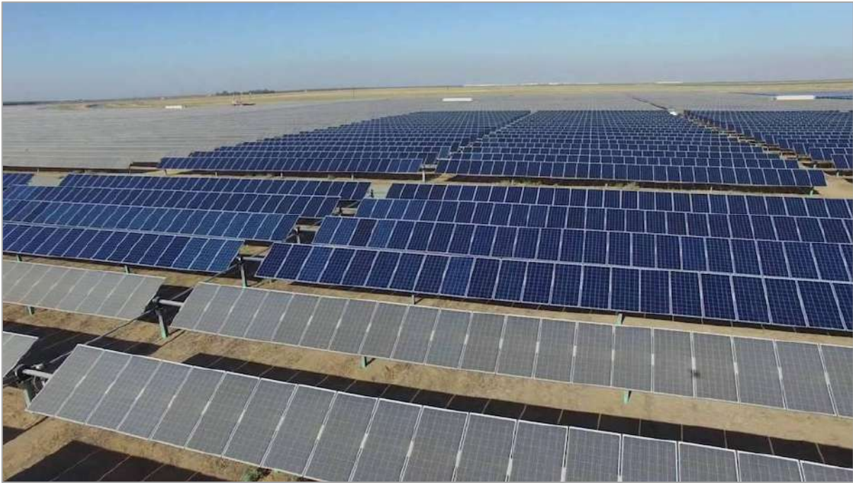
Figure 14: Example of roads between trackers and medium voltage substations (source: https://ecoinventos.com/ )
