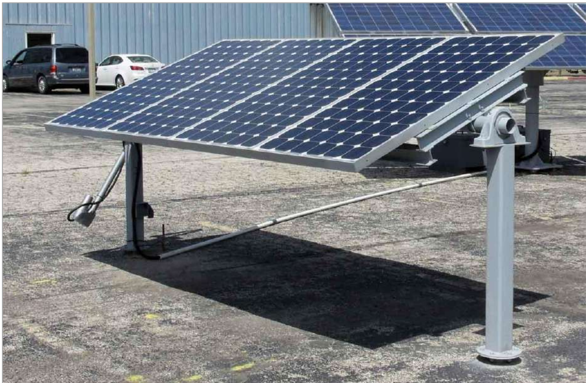
Figure 10: Example of PV Module mounted on a Single Axis Tracker
