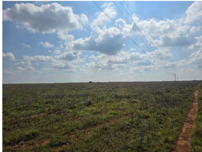
Figure 61: The existing powerline that traverses the Project Site
