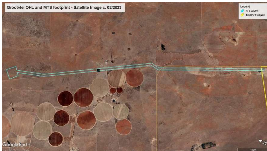
Figure 21: Historical satellite image (Google Earth) dated c. 2023 of the OHL corridor and MTS area (blue polygon) showing agricultural fields adjacent to the northern section and within the southern section
